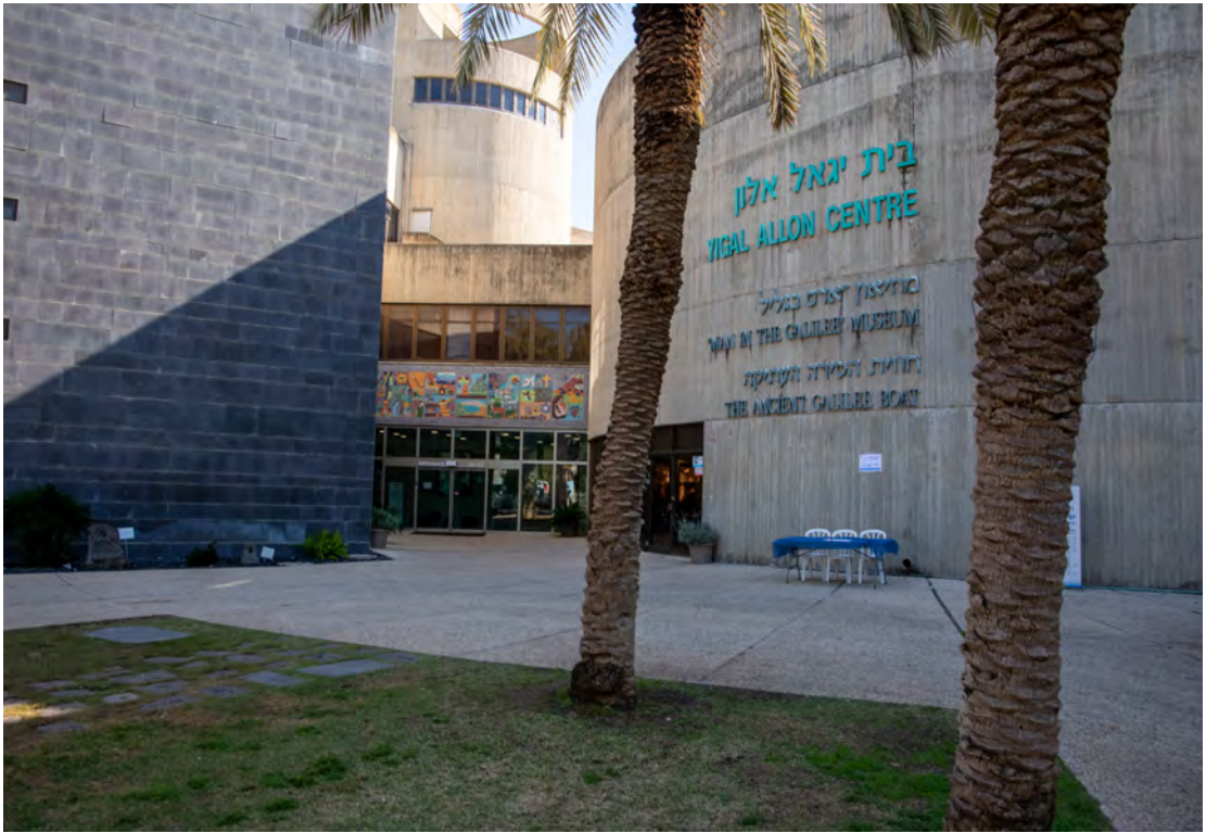
VIEW SOUTHEAST: THE YIGAL ALLON CENTER HOUSES THE GALILEE BOAT, A MUSEUM (SEE BELOW), AND AN EXHIBITION CALLED THE SANHEDRIN TRAIL.
